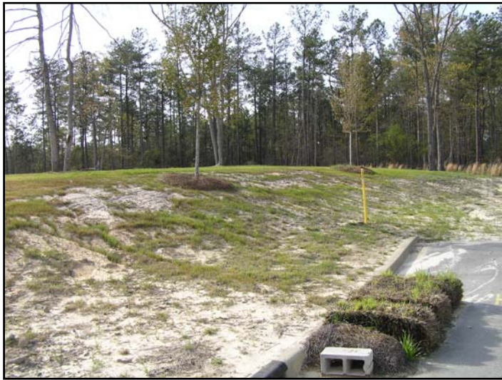
Looking @ Phase 2 from Phase 1
