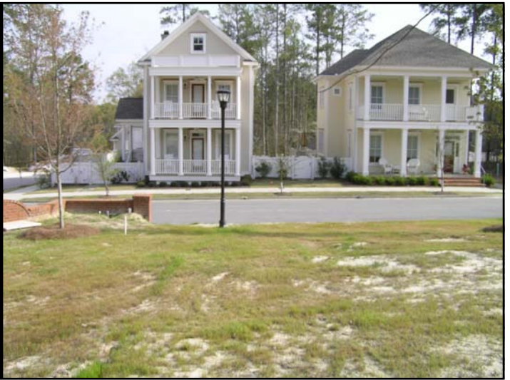
Looking @ Phase 1 from Phase 2
